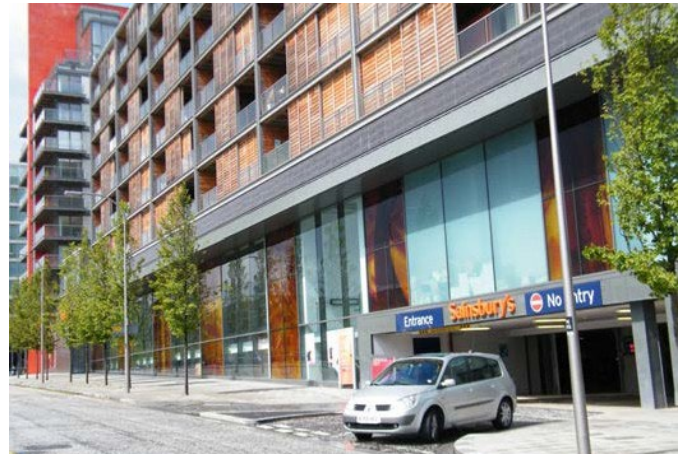
Integrated parking solution (Vizion Development, CMK) where the car park entrance is kept to a minimum and designed as part of building facade
