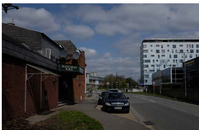
Duncombe Street looking north to Brunel roundabout
