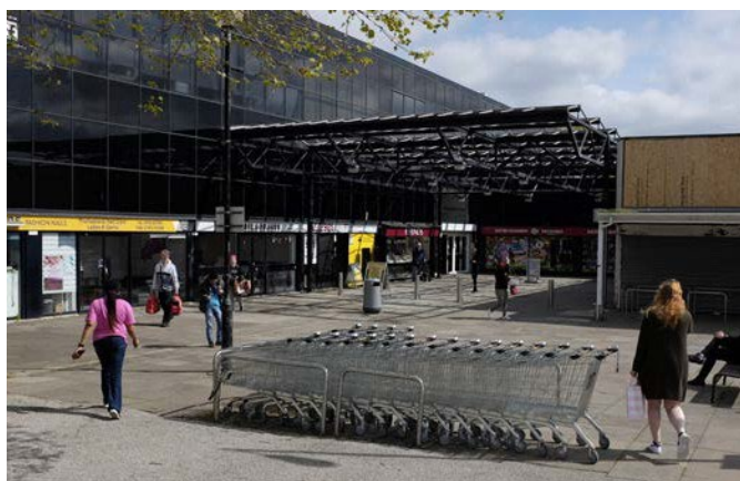
Entrance to Brunel Centre from former Sainsbury’s store car park
